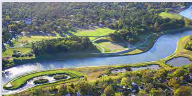
Figure 13. Designed to reduce the risk of flooding, the Brays Bayou Flood Damage Reduction Project includes wetland creation to collect stormwater and improve water quality. Photo courtesy of HCFCD.
