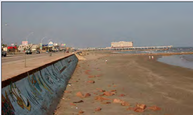
Figure 7. Galveston Seawall (2005). Source: Bob McMillan, Federal Emergency Management Agency.
